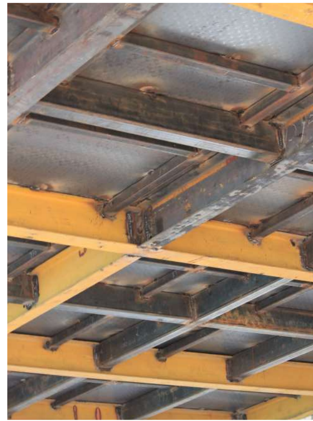
PREFAB METAL STRUCTURAL/FLOOR WORK
